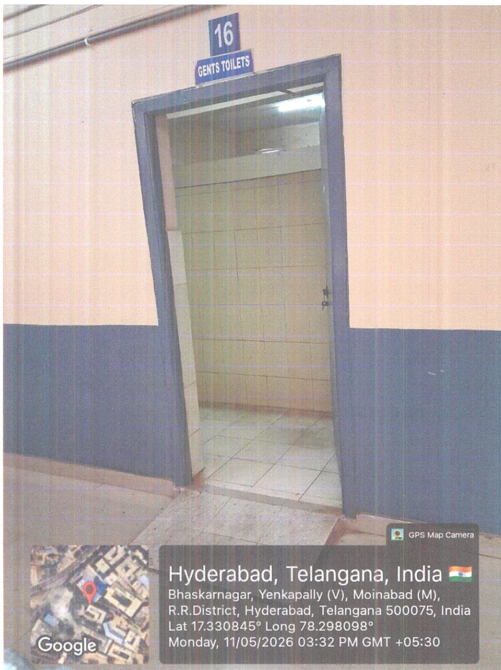
Fig. 6: Ramp towards Gents Toilet
