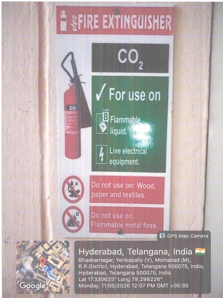
Fig. 13: Caution Sign Board
