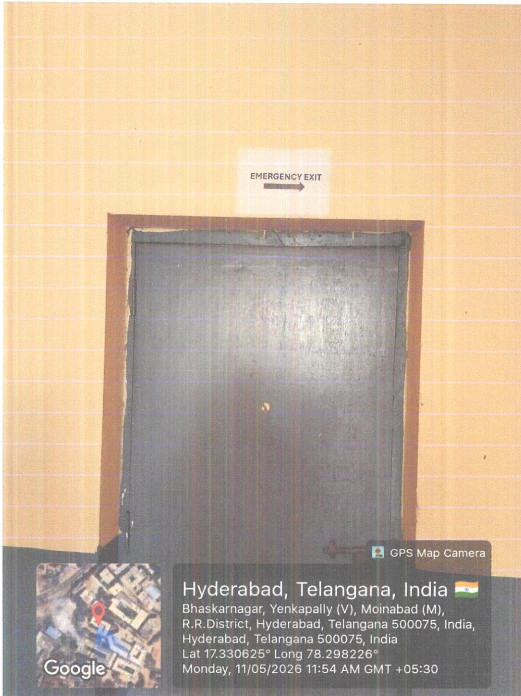
Fig. 17: Sign Board Showing Exit in case of Emergency
